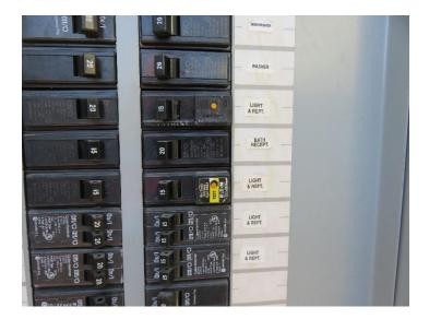
> The left side center bedroom electricals lack wiring to a fire safety AFCI safety breaker.
