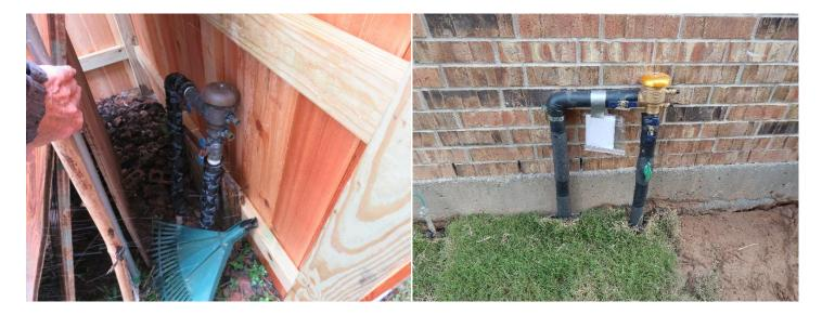
The backflow preventer should have an intermediate shut off valve on the supply side.
