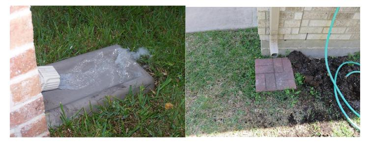
➤ Drainage at the left side of the home is not installed to allow for proper drainage. Improved drainage is needed.
