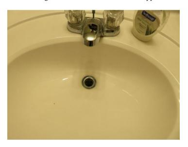
> The left sink in the Master bathroom lacks a functioning stopper.
