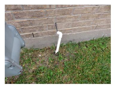
> The sprinkler system appears to lack a rain sensor that acts as an automatic shut-off during rainy and wet periods.
