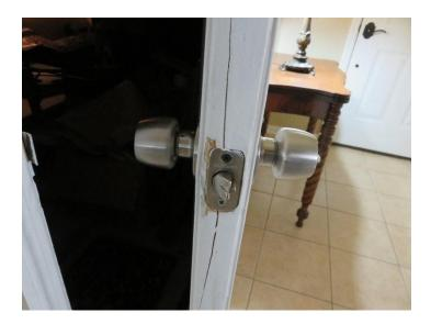
> The rear entry door displays a cracked door jamb, rust, damaged trim and damaged exterior adornment.
