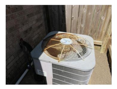
The AC condensing unit documents that the maximum circuit breaker amperage to be used is 30 AMP. The breaker in the main service panel for this unit indicates that there is a 35 AMP breaker in place.
