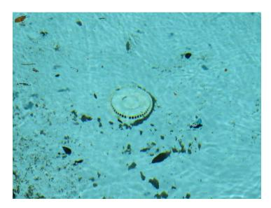
> The pool drain is required to terminate in a sanitary drain/system. Draining pool water to the street or in the current installation to the left side lawn is prohibited.
