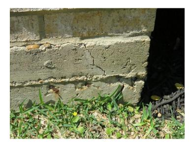
➤ Post tension foundation cable ends about the home are exposed. Allowing these cable ends to remain exposed to moisture and weather elements could eventually cause the cable to weaken and possibly lose strength. Evaluation by a professional foundation contractor familiar with decay of post tensions cables may be required. All exposed cable ends should be properly covered/protected to prevent further deterioration.
