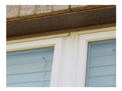
Exterior window sills are required to be installed to slope at least at a 15\* angle away from the home/window to properly drain/shed water away from the home.
