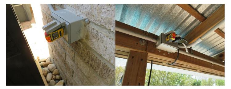
➤ The outlet at the rear upper patio wall is a GFCI apparatus but the weather cover is installed upside down.
